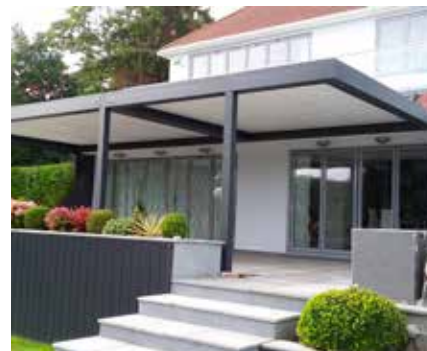
Possibility to have overhang up to 2 m and up to max. 1/3 of the surface
