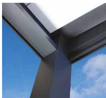
Water drainage through the gutters directly in vertical posts
